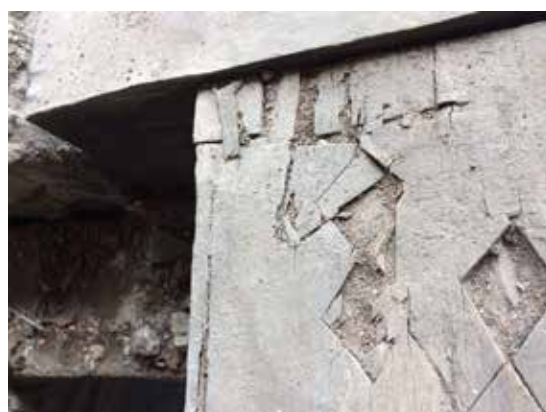
Figure 4. Southwest direction structural connection marker.
